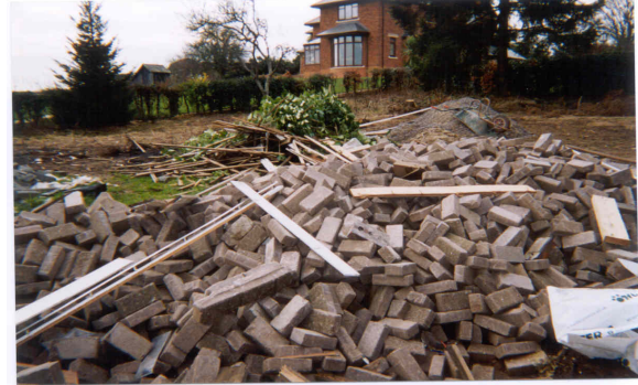
Figure 3 Reclaimed paving bricks for reuse
