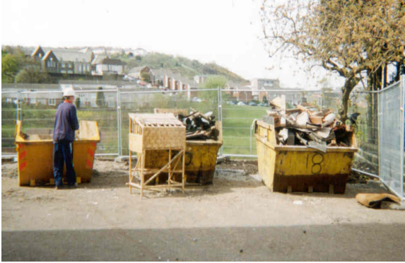
Figure 2 Segregation of waste on site after introducing waste minimisations techniques
