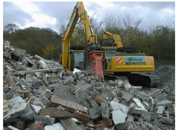
Figure 1 Crushing rubble for reuse
