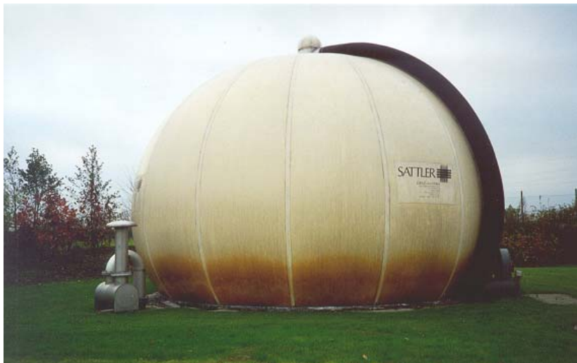
Plate 5.5 Anaerobic Digestion Plant
