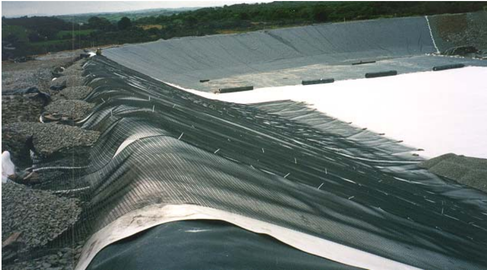
Plate 5.6 An Engineered Landfill Site Under Construction
