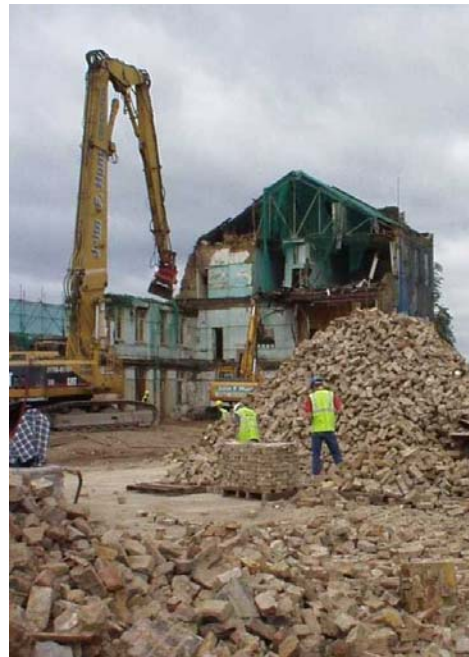
Figure 5.1 Demolition & Segregation of Bricks ( Courtesy of Channel Tunnel Rail Link )
