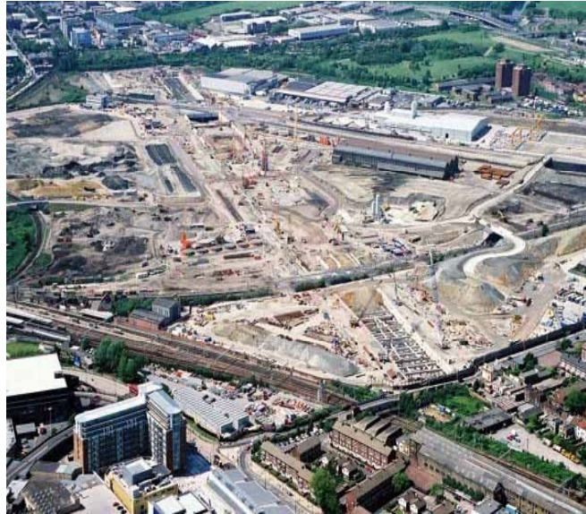
Fig. 3.1. Aerial View Of Construction Work On The CTRL Project
