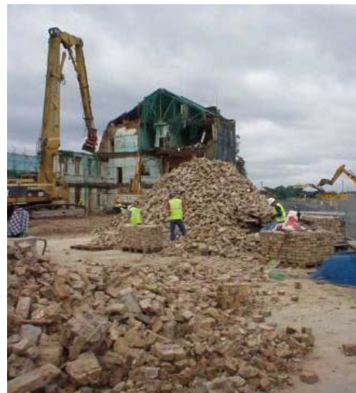
Figure 3. Segregation of demolition material on the Channel Tunnel Rail Link project
