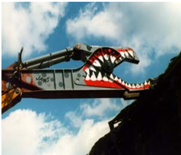
Figure 7.1 Jaw Crusher With Long Reach Crane To Remove Upper Part Of Building.
