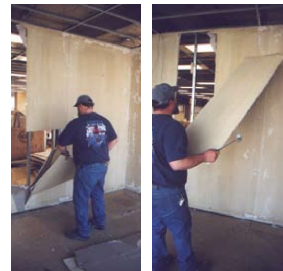
Plasterboard dismantling
