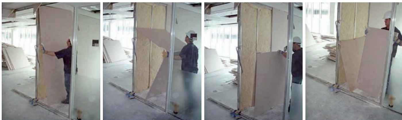
1 Dismantling plasterboards
