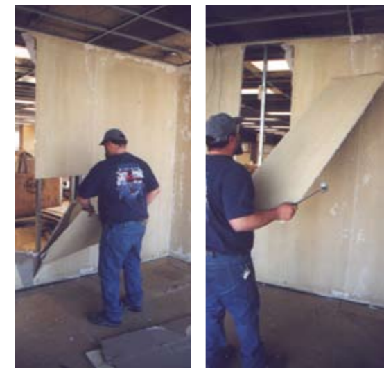
Plasterboard dismantling
