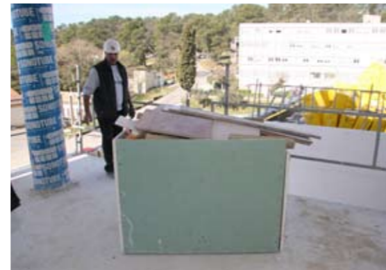
Plasterboard sorting
